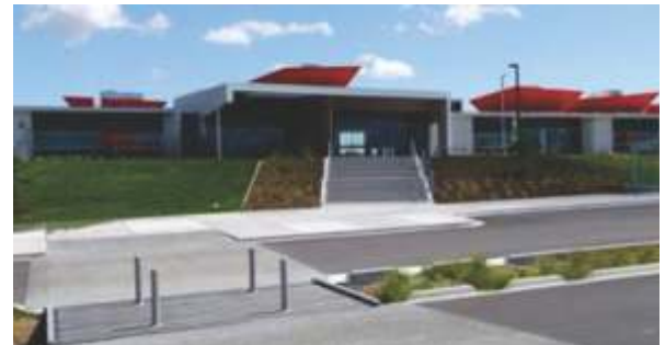
Hobsonville Point Primary School
